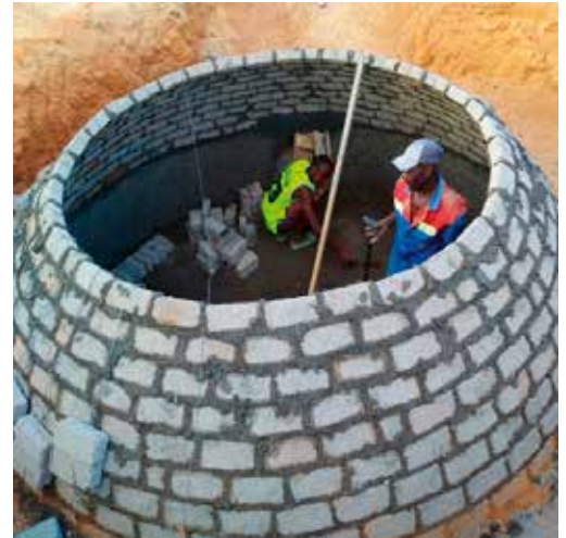
TVET students constructing a biogas digester.
